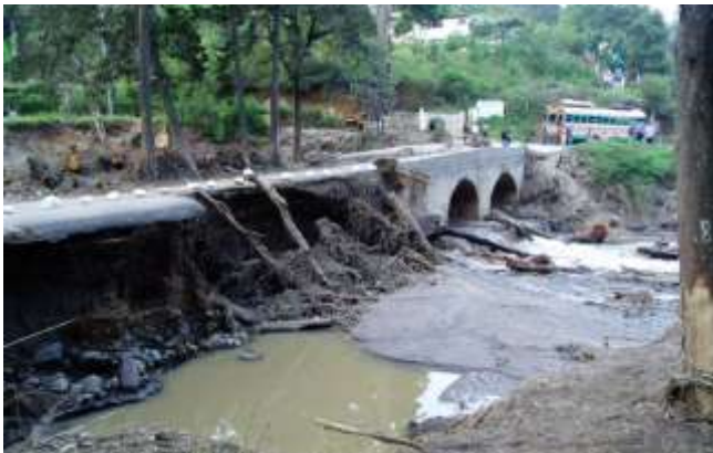
Picture from Madre Ana Maria shows the road washed out near Patzún
